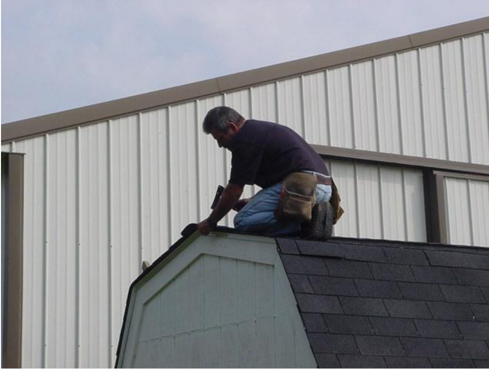
Marty Lien putting the finishing touches on the roof.
